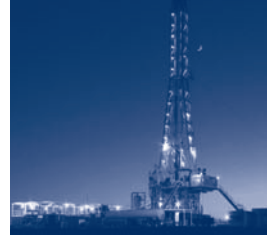
The Weatherford Rig # 828 (Le Tourneau Technologies Inc.) is being built in Dubai and expected to be delivered to Australia in January 2009.
